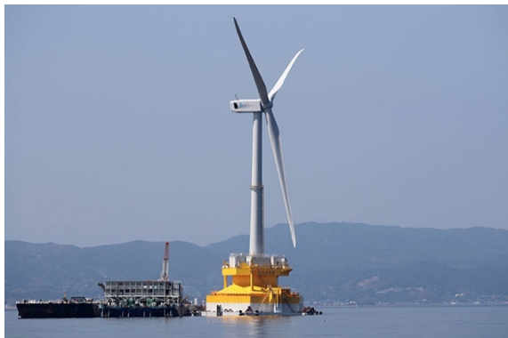
Figure 1 - Photo of a FOWT being installed at Fukushima's coast.
